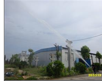
Photo of fire safety equipment check the fire hydrant.JPG
